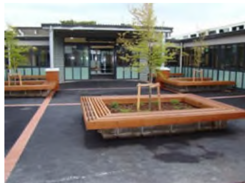
Wellington College Technology Block upgrade Before and after gallery
